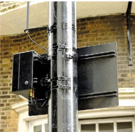
**LEFT:** The zone controller covers a number of sensors and can be mounted on any convenient post
